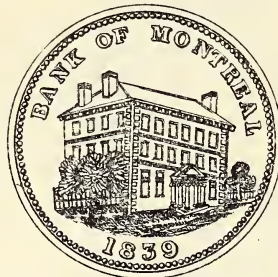
Front and side view of building.
